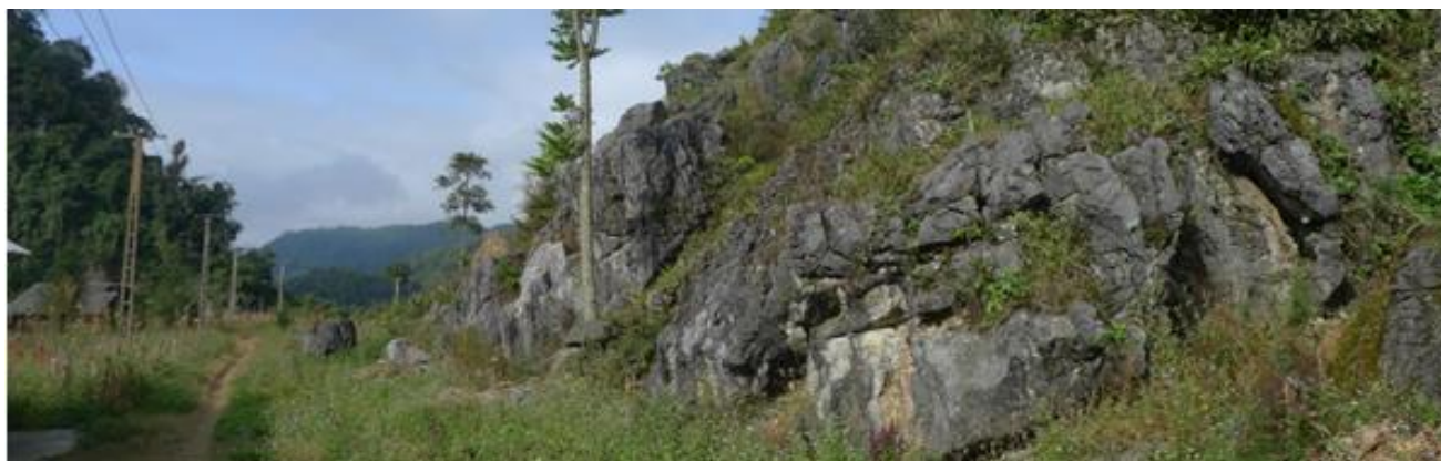
Picture 22: Electric line running beside a village path
