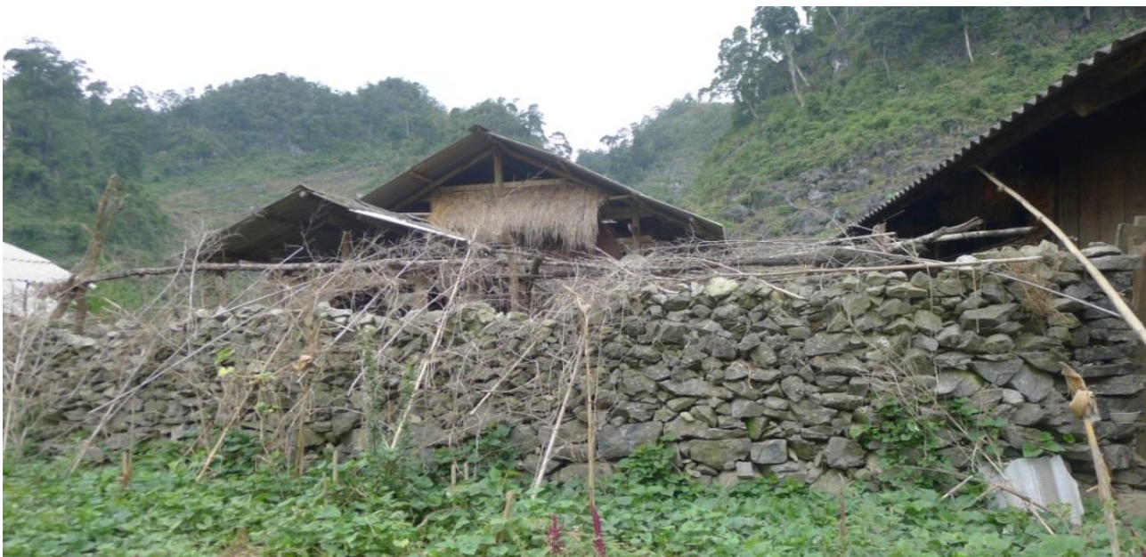
Picture 13: A house with a stone wall
