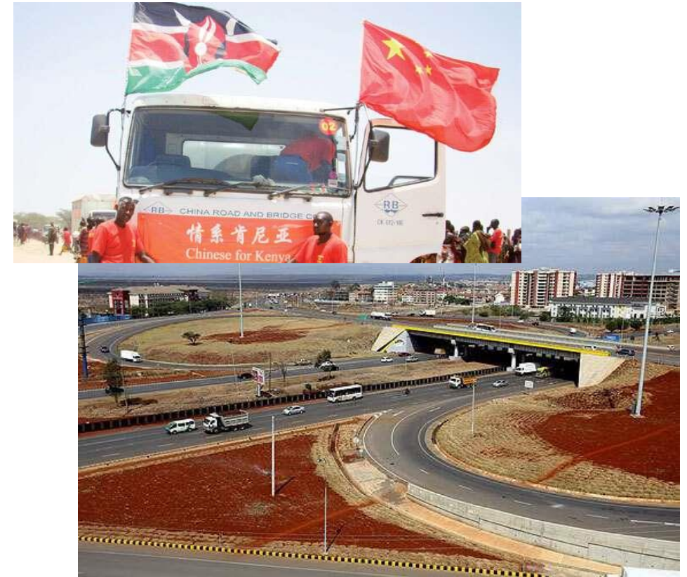
Nairobi Eastern Bypass built by CRBC, Kenya
